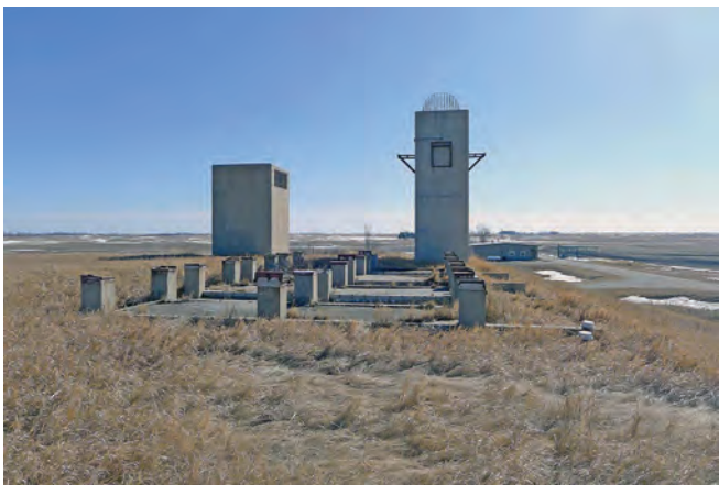
Pads for RLOB AC condensers foreground, air intake shaft left, exhaust stack right
